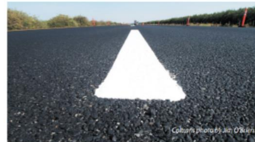
A section of new-generation road striping was recently laid on Interstate 5 near Orland, about two hours north of Sacramento.
